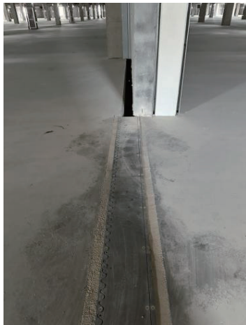
Movement Joints (Settlement)
