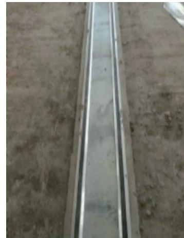
Movement Joints (Seismic)
